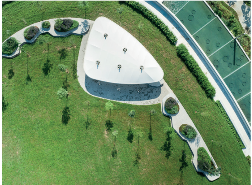
The Keppel Marina East Desalination Plant is Singapore's first and only large-scale dual mode plant which can treat both seawater and reservoir water.
