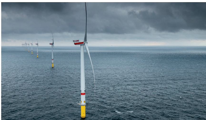
Located 59 km off the coast of Lower Saxony in the North Sea, Germany, Borkum Riffgrund 2 is an offshore wind farm with an operating capacity of approximately 465 MW.
