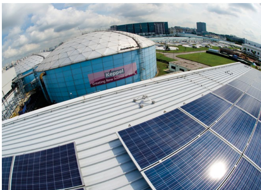
The solar photovoltaic installation at Keppel Seghers Ulu Pandan NEWater Plant produced approximately 1,100 MWh of energy in 2013.
