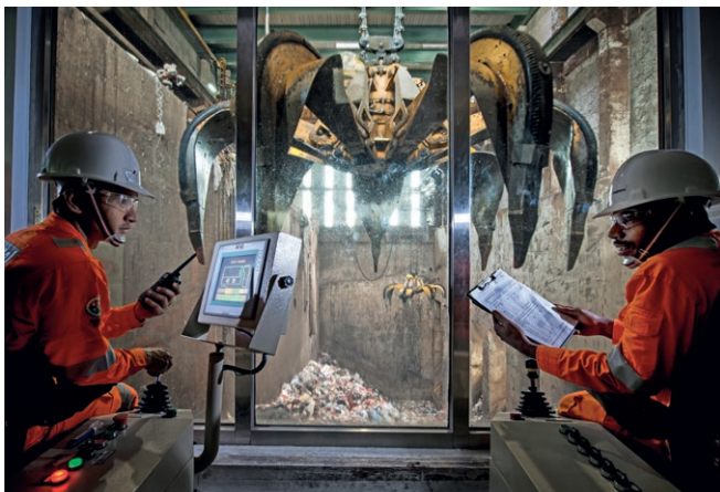
Both WTE plants consistently meet and exceed requirements in their Incineration Services Agreements.
