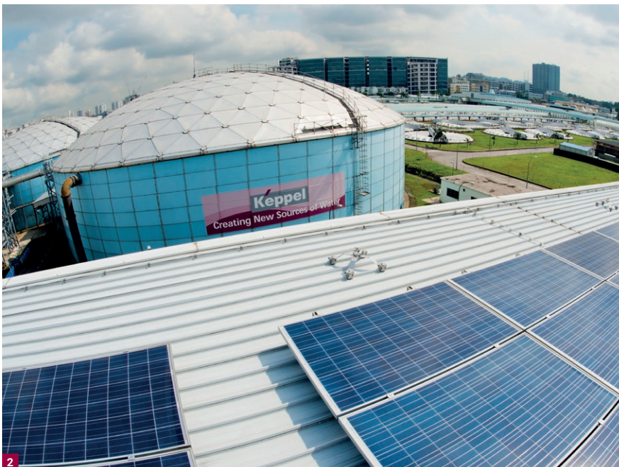
1 Several of KIT's assets are Key Installations in Singapore as they provide essential infrastructure services, like electricity from Keppel Merlimau Cogen (pictured).
