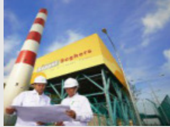
Tuas DBOO Plant
