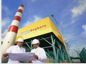
Tuas DBOO Plant
