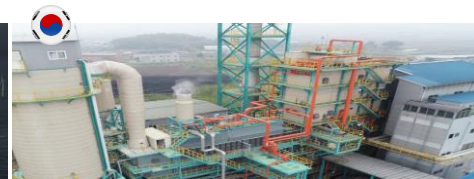
EMKH – Integrated Waste Platform 1
