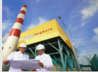
Tuas DBOO Plant
